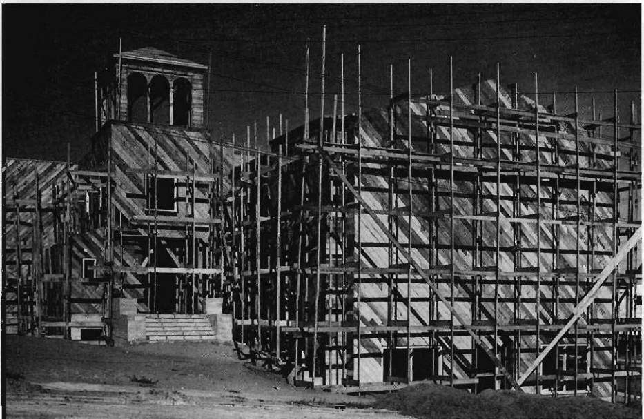
Sunset Ward Chapel under Construction in 1939.
